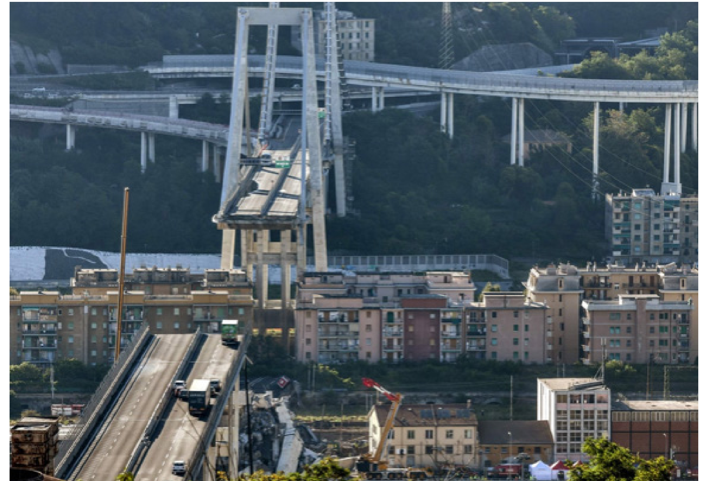
The mother of infrastructure failure: Morandi bridge collapse in Genoa, Italy, 2018
